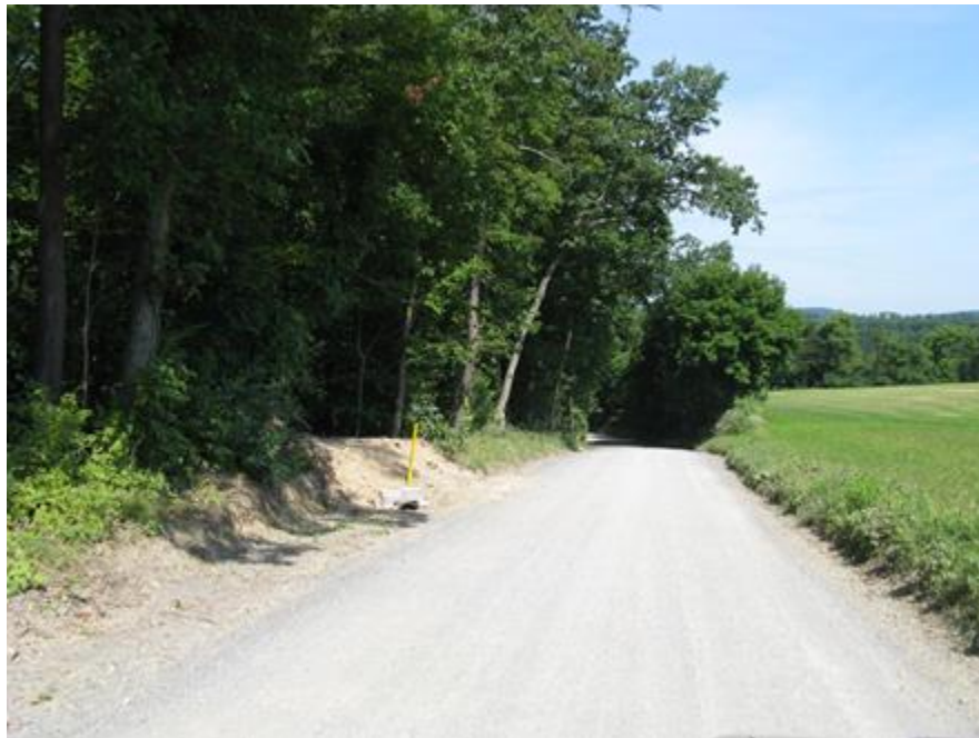
Above: A section of Shaffer Hill Road improved inside Washington Township during 2012.
