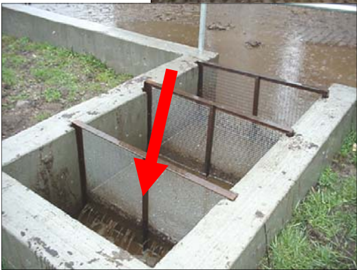
A screen box (left and below left, different operations) filters manure solids that flow from an improved barnyard during a rain event. The first screen (below left) prevents heavy solids from entering the screen box. The second and third screens have smaller spaces that filter smaller solids. Notice the water flowing from the final screen marked with a red arrow (left). This water flows into a concrete septic tank where the water settles, then is siphoned or pumped to a vegetative filter area. Regular cleanout maintenance is needed for this BMP to work to its fullest capacity.
