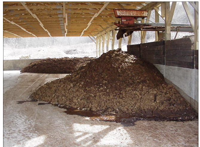
Manure can enter roofed manure stacking structures either by gutter cleaner from the stanchion barn (above) or through a tractor push-off ramp (with tractor guard) from the barnyard (left).
