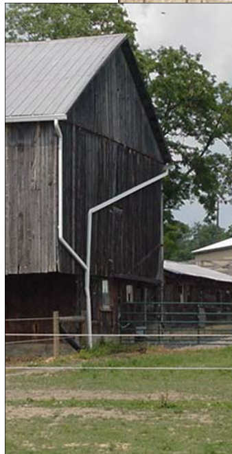
Roof runoff being diverted away from a concrete barnyard on two separate dairy farms (top two photos) and a horse pasture on another farm (center photo). Example of roof gutters and downspouts installed on a roofed ACA far (left) and a composter attached to a poultry manure storage (below)..
