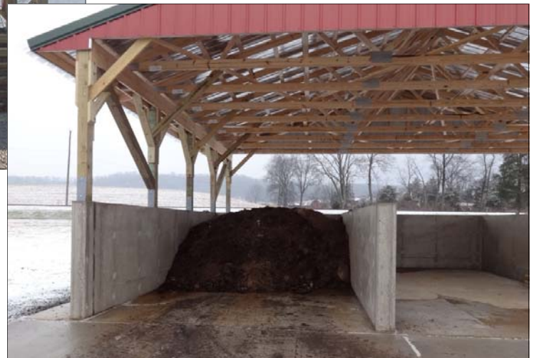
Stand alone poultry mortality composting structures constructed with treated lumber (left) and concrete walls (below).
