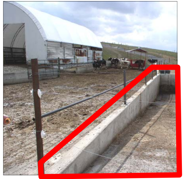
The barnyard shown on the center right photo utilizes a concrete settling basin (outlined in red) to filter manure laden water before it is screened and pumped to a filter area in one of the nearby pastures (not shown)
