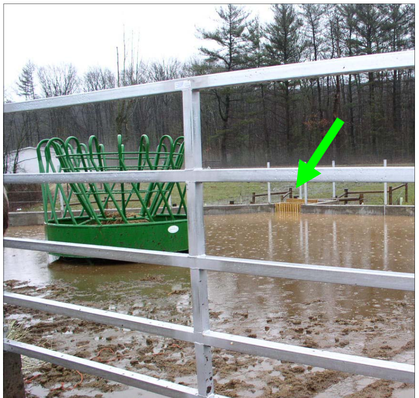
Two photos (right and bottom, next page) show how a properly designed improved barnyard should work during a rainstorm. The water laying within the barnyard indicates that the floor is sloped towards the screen box (green arrow, right photo) and the concrete curbs contain and hold the stormwater and do not allow it to leave the site (right photo and next page's bottom photo).
