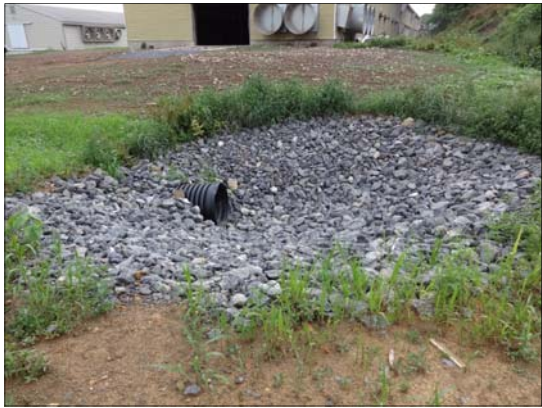
An example of a rock lined inlet diverting water away from poultry facility (above left). An outlet pipe taking stormwater to a drop box (above right)
