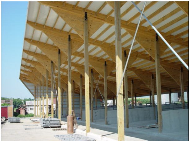
Although not funded by any public financial assistance grants, this farmer installed netting and a type of monoslope roof that prevents starlings from roosting in his roofed ACA (left and above).
