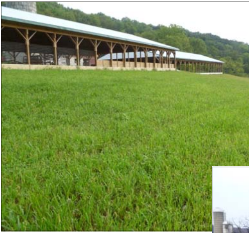
Vegetation along manure BMP sites (top three) where earth was disturbed during construction.
