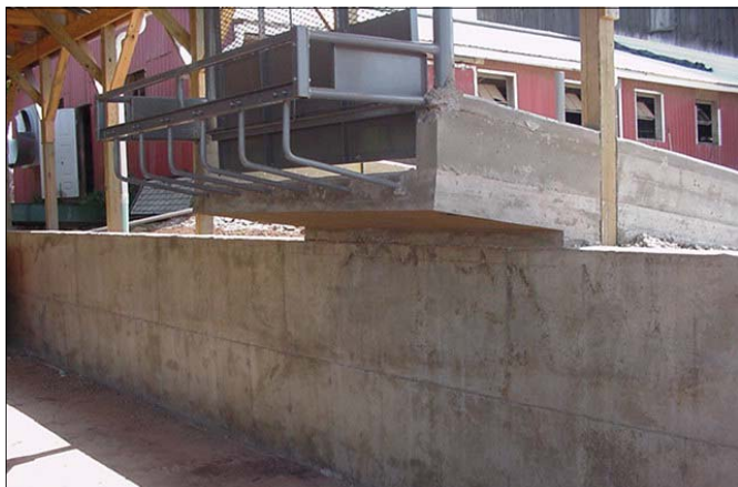
Roofed manure storage stacking structures with concrete walls constructed to store dry stackable manure (right and below).
