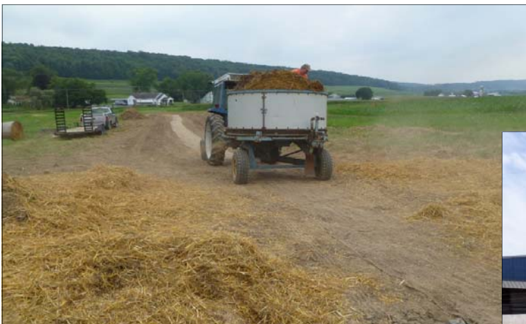
When the project is almost completed, no matter if it is a grassed waterway (left) or an improved barnyard (below), establishing vegetation to keep the soil in place is critical. Mulching is necessary to protect the seed and maintain soil moisture during early vegetation growth.
