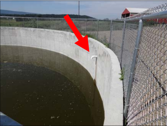
Liquid manure storage concrete tank constructed to store not only manure but also milkhouse wastewater from a pipe (above, see red arrow) or collected barnyard water from a pipe (right, see yellow arrow).
