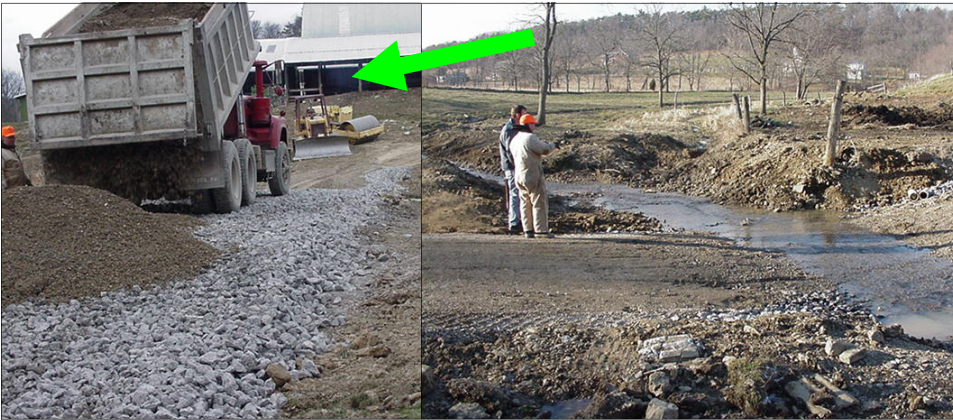
Above photos show an excavator, in coordination with NRCS staff, build a cattle walkway and stream crossing for a dairy farm. Notice the different types of stone used. The arrow points to the vibratory roller needed and bulldozer.
