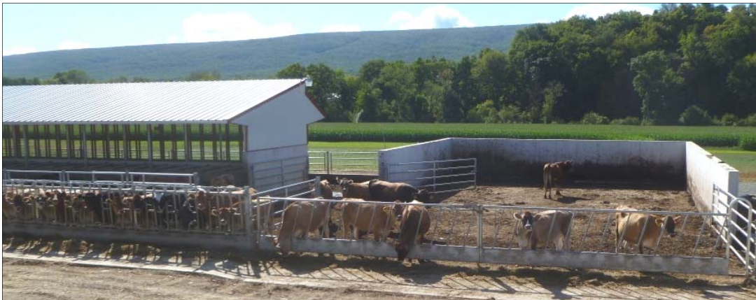
An unroofed manure stacking area with concrete walls serving a concrete cattle barnyard and lot. (left)
