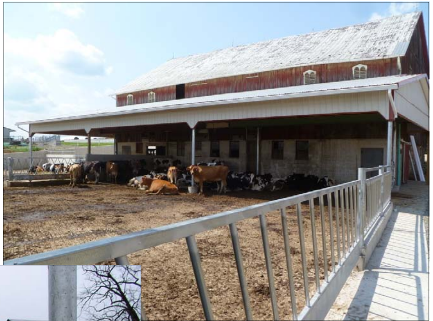
A combination of an open and roofed barnyard/ACA. Notice the roof runoff controls (above).
