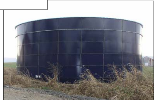
Typically, liquid manure storages have pads where portable manure pumps can be placed (left). Farmers have also installed liquid manure storages made of metal (right).
