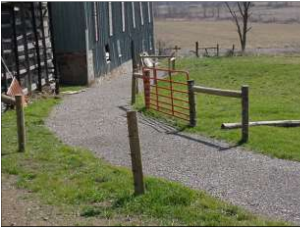
Example cattle walkways at two separate farms (above and left). Geotextile may be needed at some places due to soil type and nearness to streams.
