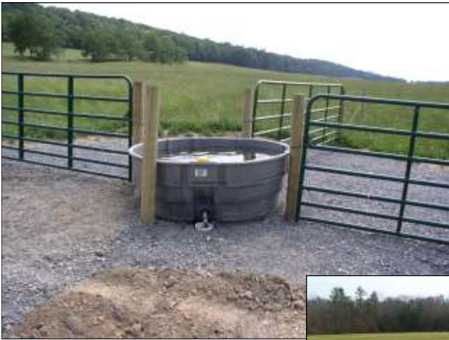
Reinforced gravel pads placed around newly installed water troughs and waterers at various beef and equine operations (left, right, below and right).
