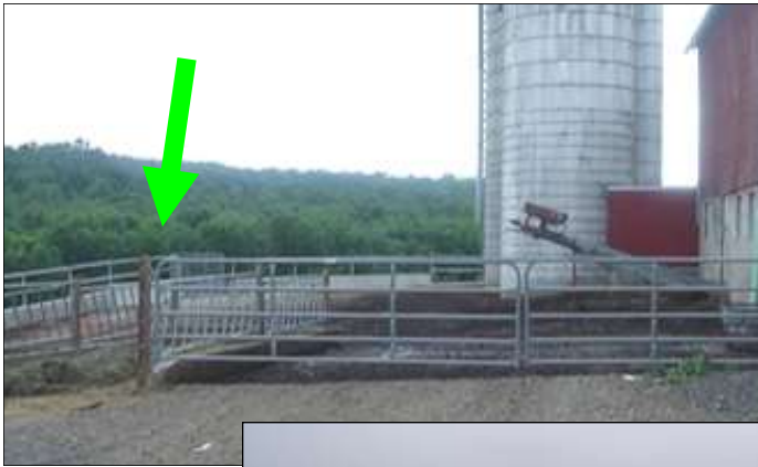
The dairy farmer (left) had improved his existing barnyard. This allows him to feed his cattle and transfer manure directly into a manure spreader with an existing gutter cleaner or a newly installed push off ramp (green arrow). The farmer below connected a newly improved barnyard with a liquid manure storage via push off ramp (yellow arrow).
