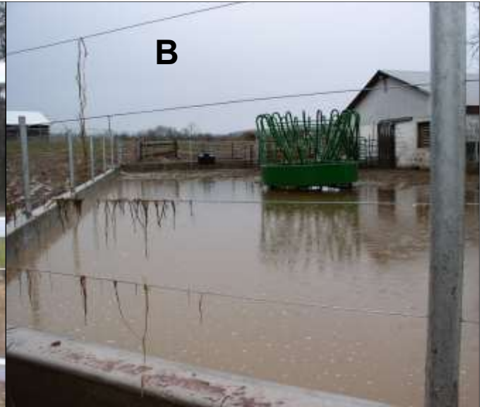
Two photos (“A” and “B” on this page) show how a properly designed improved barnyard should work during a rainstorm. The water laying within the barnyard indicates that the floor is sloped towards the screen box (green arrow, A photo) and the concrete curbs contain and hold the stormwater and do not allow it to leave the site (photos A and B).
