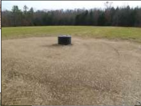
Reinforced gravel pads placed around newly installed water troughs and waterers at various beef and equine operations (left, right, below and right).
