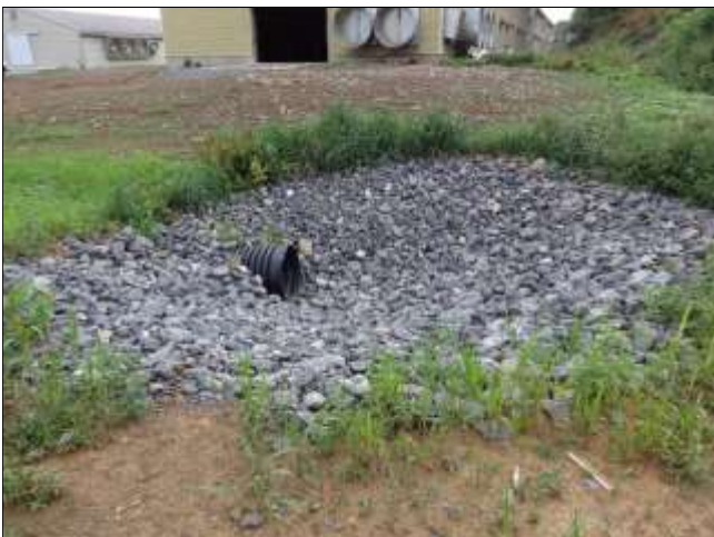
An example of a rock lined inlet diverting water away from poultry facility (bottom left). An outlet pipe taking stormwater to a drop box (bottom right)
