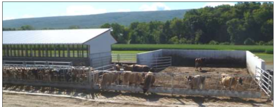
An unroofed manure stacking area with concrete walls serving a concrete cattle barnyard and lot. (bottom)
