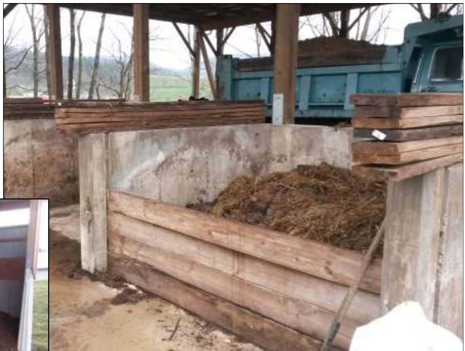
Four examples of mortality composting bins as part of roofed poultry manure stacking structures on different farms. One has walls of treated lumber within the manure storage (above left), one has walls of treated lumber as an extension of the manure storage (above right), one has poured concrete walls (center right) and one has bins separated by precast concrete walls (below left).
