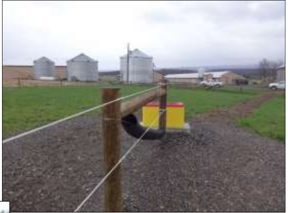
Reinforced gravel pads placed around newly installed water troughs and waterers at various beef and equine operations (left, right, below and right).
