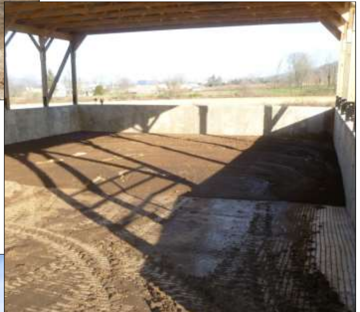
Roofed manure storages with concrete walls for various management situations. Top left photo: Dairy stackable manure from a gutter cleaner and a nearby barnyard. Top right photo: Liquid dairy manure scraped from alleyways regularly into a roofed storage to limit additional rainwater. Second from bottom: Roof installed over existing concrete manure stacking area for a beef herd barnyard.
