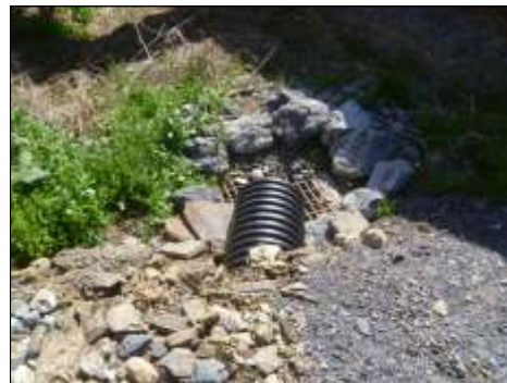
An example of a rock lined inlet diverting water away from poultry facility (bottom left). An outlet pipe taking stormwater to a drop box (bottom right)
