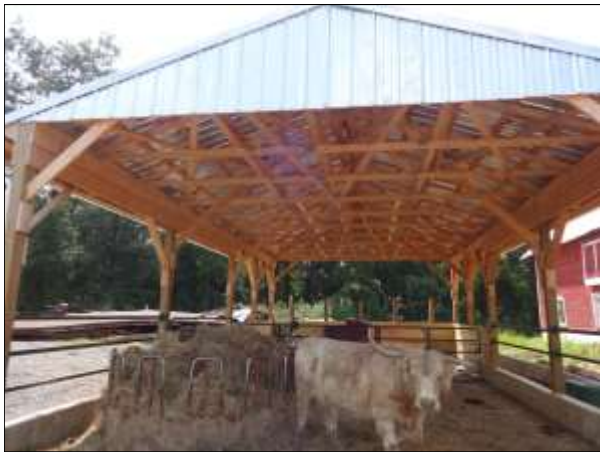
A stand alone roofed barnyards/ACAs structure (top right photo) and a barnyard/ACA with a roof extended from the main barn (center photo).
