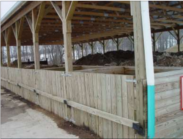
Four examples of mortality composting bins as part of roofed poultry manure stacking structures on different farms. One has walls of treated lumber within the manure storage (above left), one has walls of treated lumber as an extension of the manure storage (above right), one has poured concrete walls (center right) and one has bins separated by precast concrete walls (below left).
