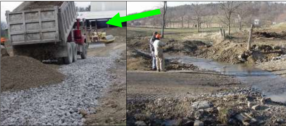
Above photos show an excavator, in coordination with NRCS staff, build a cattle walkway and stream crossing for a dairy farm. Notice the different types of stone used. The arrow points to the vibratory roller needed and bulldozer to complete the job.
