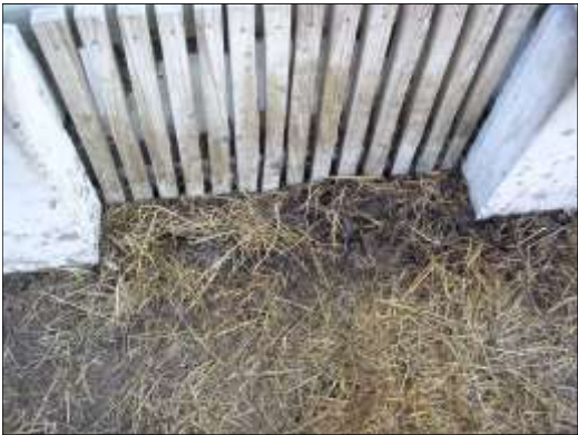
A screen box (center left and center right, different operations) filters manure solids that flow from an improved barnyard during a rain event. The first screen (center left) prevents heavy solids from entering the screen box. The second and third screens have smaller spaces that filter smaller solids. Notice the water flowing from the final screen marked with a red arrow (center right). This water flows into a concrete septic tank where the water settles, then is siphoned or pumped to a vegetative filter area. Regular cleanout maintenance is needed for this BMP to work to its fullest capacity.
