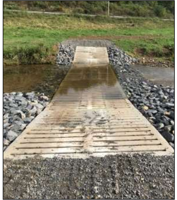
In pastures, streambank fencing go hand in hand with cattle stream crossings.
