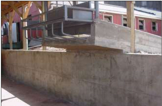
Roofed manure storage stacking structures with concrete walls constructed to store dry stackable manure (bottom two photos).
