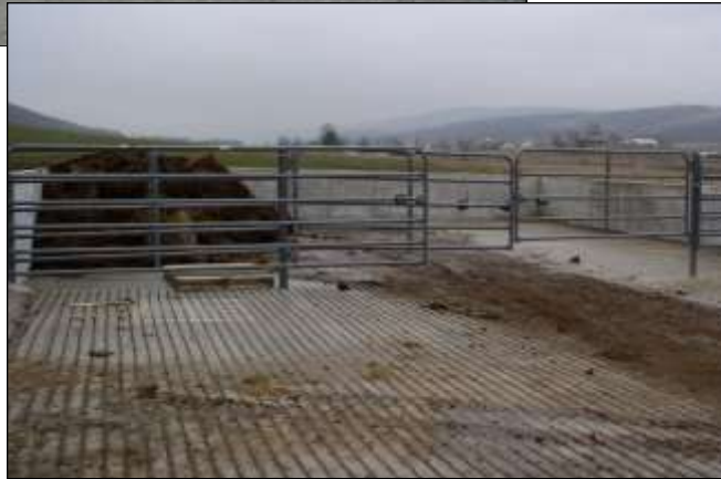
A farmer can utilize a manure storage stacking area connected to an improved barnyard. This beef farmer has a manure storage stacking area with 4 ft. concrete walls and floor (left).
