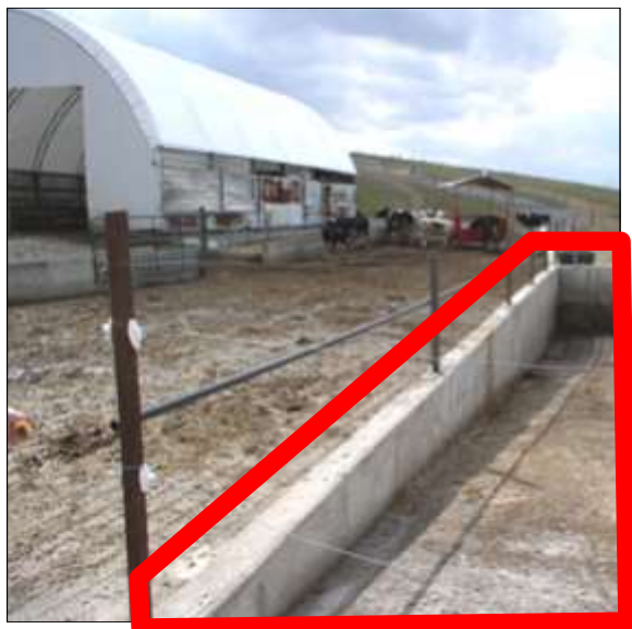
The barnyard shown on the bottom left photo utilizes a concrete settling basin (outlined in red) to filter manure laden water before it is screened and pumped to a filter area in one of the nearby pastures (not shown)
