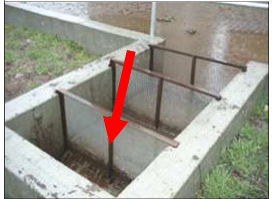
A screen box (center left and center right, different operations) filters manure solids that flow from an improved barnyard during a rain event. The first screen (center left) prevents heavy solids from entering the screen box. The second and third screens have smaller spaces that filter smaller solids. Notice the water flowing from the final screen marked with a red arrow (center right). This water flows into a concrete septic tank where the water settles, then is siphoned or pumped to a vegetative filter area. Regular cleanout maintenance is needed for this BMP to work to its fullest capacity.
