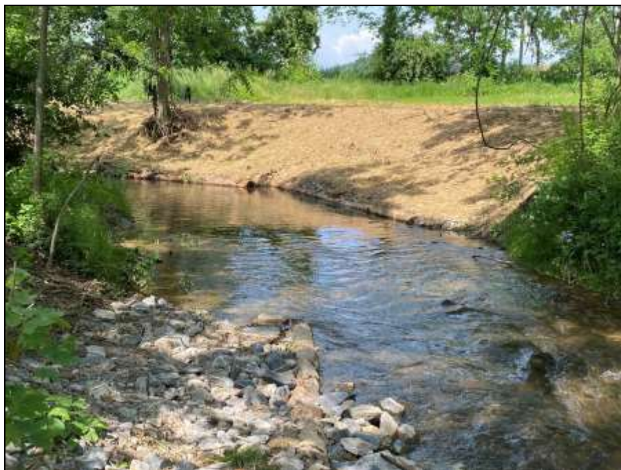
A mudsill carefully excavated, seeded and mulched along a streambank (bottom photo). Notice the supporting logs and stone installed.
