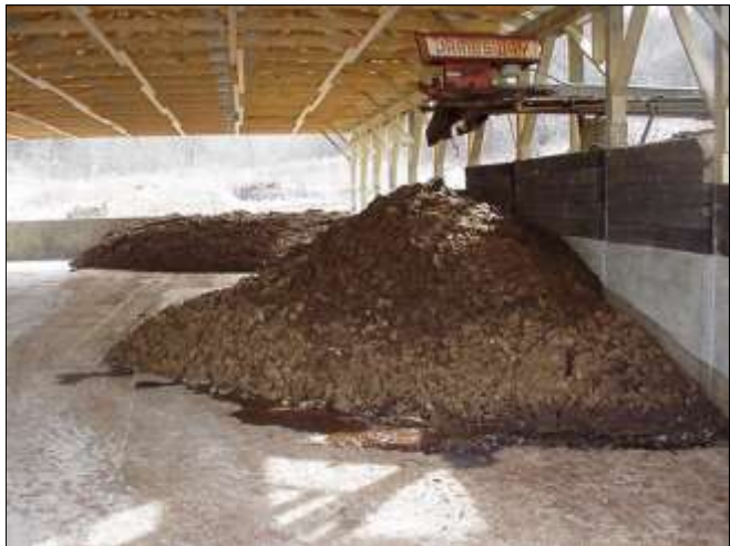
Manure can enter roofed manure stacking structures either by gutter cleaner from the stanchion barn (bottom right) or through a tractor push-off ramp (with tractor guard) from the barnyard (bottom left).
