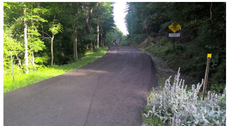
DSA placement on Long Hill Road.
