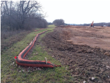
Silt sock placed at an NPDES site.
