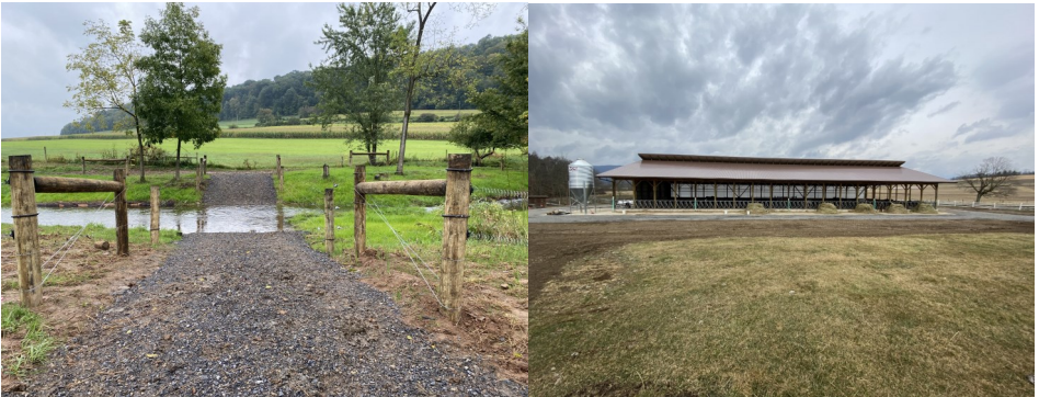
Left: Stream crossing installed along Susquehecka Creek in Franklin Township, Snyder County.
