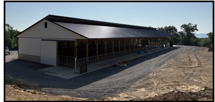
Above: Roofed Heavy Use Area (HUA) and manure storage for beef.
