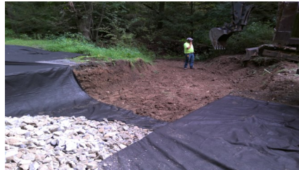
Installation of French Mattress on Covered Bridge Road, Beaver Township
