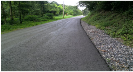
DSA Install and Drainage Improvements on Lime Road, Chapman Township
